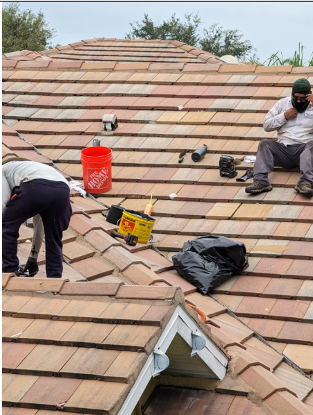
Repairs to Broken Field Tile as Well
