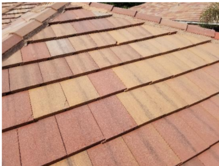
Photo 4: Tile cracking at Bldg 13
