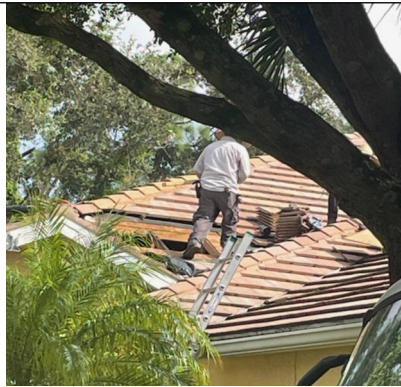
Repairs To Plywood, Truss and Roofing
