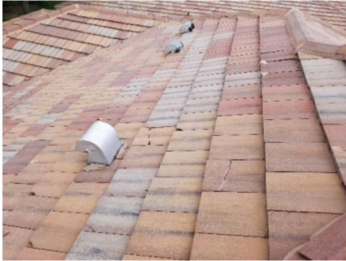
Photo 19: Cracked and shifted tile at Bldg 13
