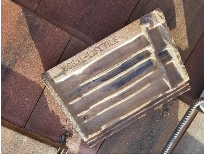
Photo 1: Existing tile – Boral Lifetile
