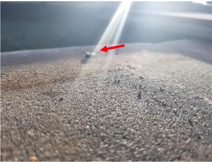
Photo 15: Fastener that doesn't appear withdrawn at Bldg 1
