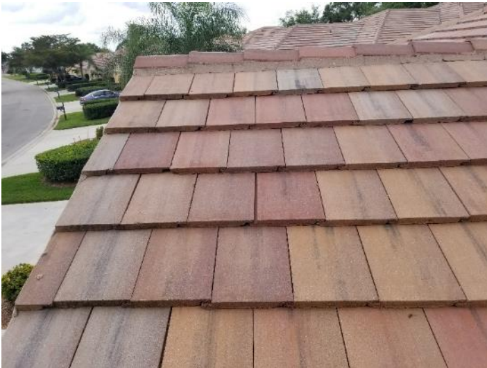
Photo 21: Tile shifting at Bldg 6
