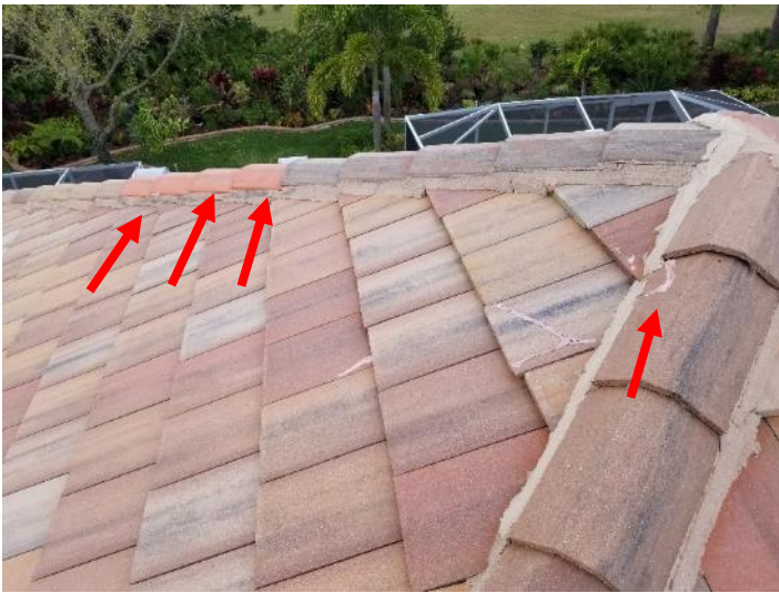
Photo 9: Cracked and mismatching hip tile at Bldg 10
