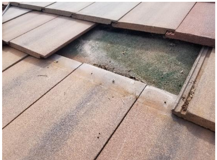
Photo 12: Fastener withdrawn & cracked tile at Bldg 27
