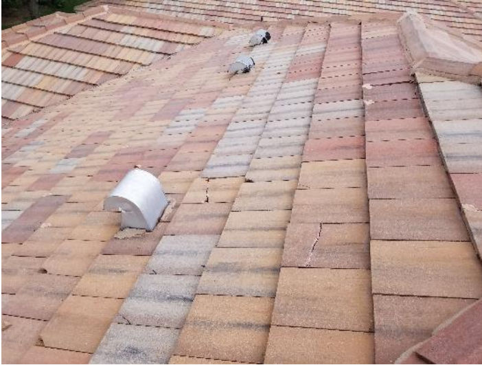
Photo 19: Cracked and shifted tile at Bldg 13
