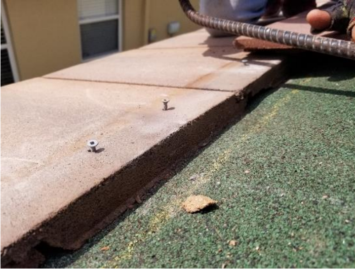
Photo 13: Fastener withdrawn & damage to fastener hole at Bldg 27
