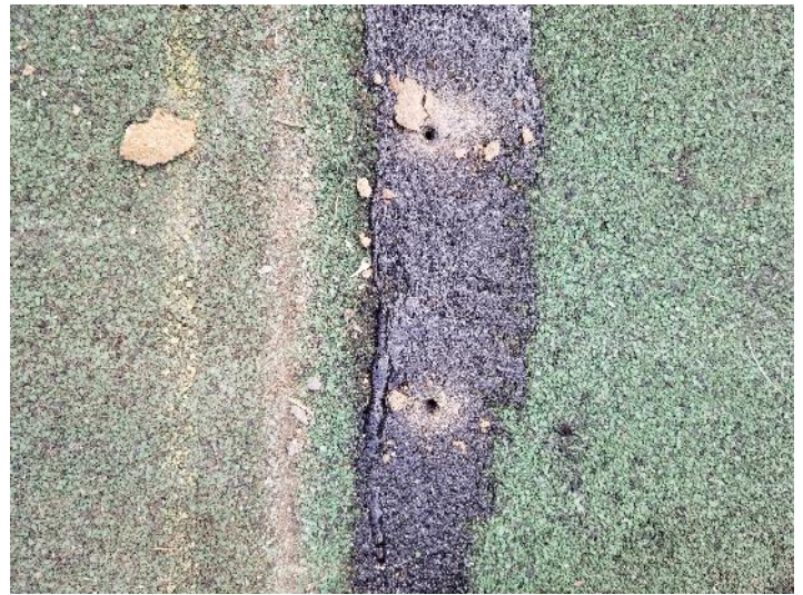
Photo 16: Undamaged underlayment at removed tile on Bldg 27
