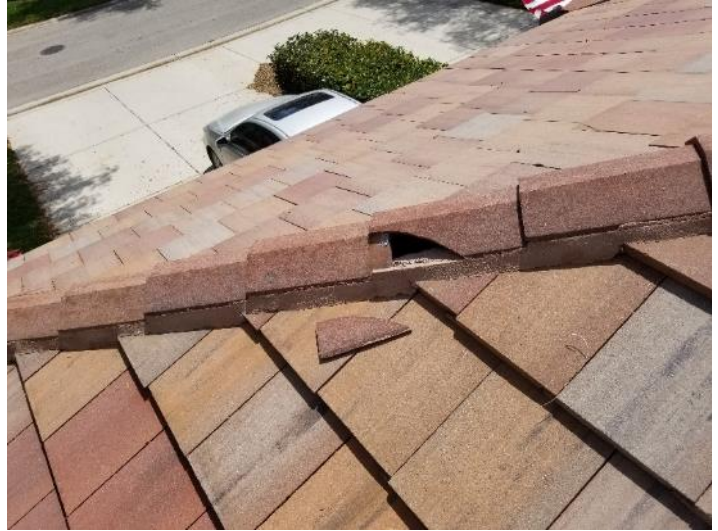
Photo 8: Cracked hip tile at Bldg 4
