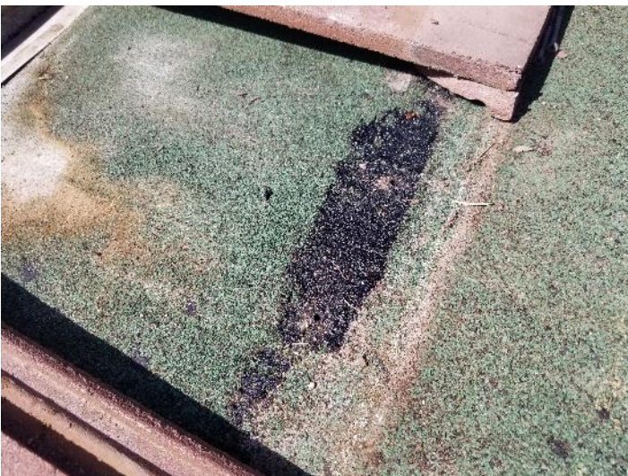
Photo 17: Undamaged underlayment at removed tile on at Bldg 11
