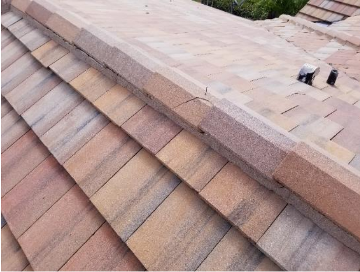
Photo 7: Cracked ridge tile at Bldg 7
