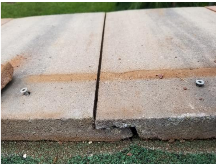
Photo 23: Tile shifting at withdrawn fastener locations at Bldg 30
