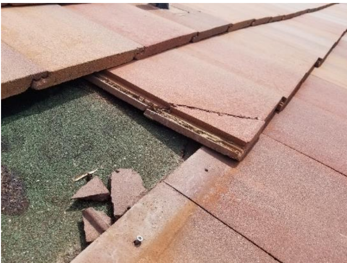
Photo 11: Fastener withdrawn & cracked tile at Bldg 21
