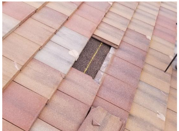
Photo 18: Cracked tile adjacent to withdrawn fasteners at Bldg 33
