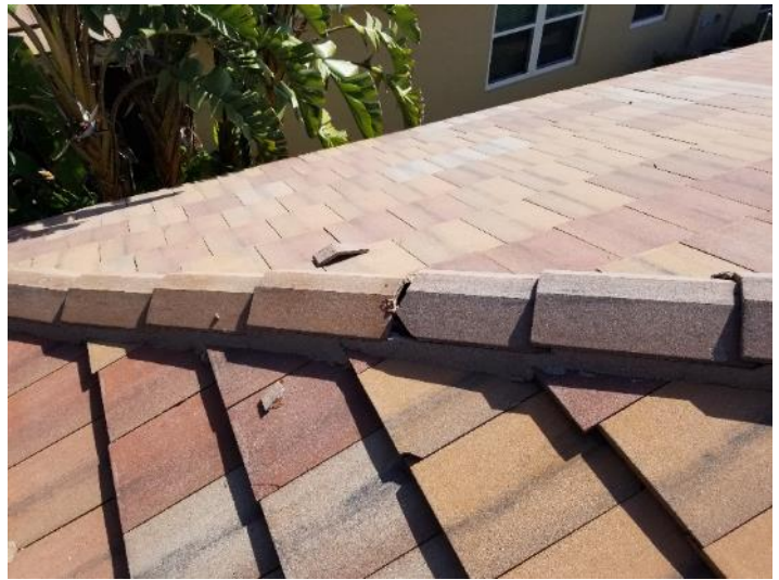
Photo 10: Cracked hip tile at Bldg 14
