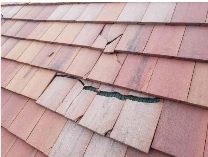
Photo 5: Tile cracking at Bldg 23
