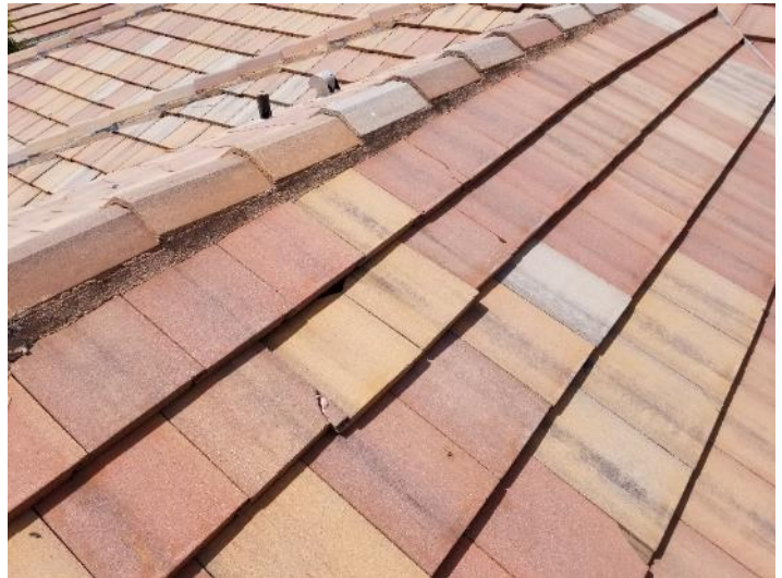
Photo 22: Tile shifting at Bldg 8
