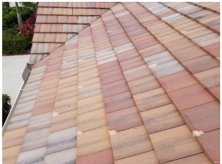
Photo 6: Tile cracking at Bldg 33
