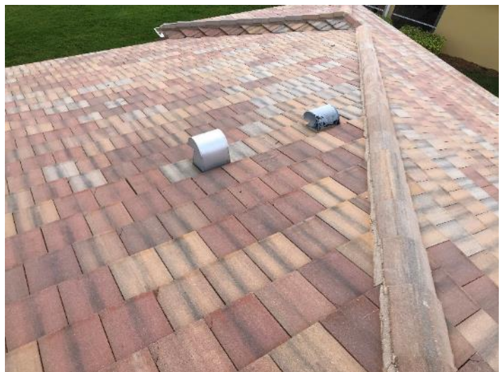
Photo 24: Tile shifting at Bldg 31
